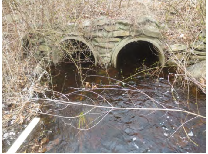
Figure 6.1.1e Somerset Reservoir Intake By-Pass Channel Outlets with Blocking Rocks
