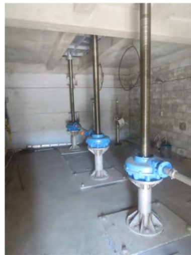
Figure 5.2.10b. 4 th Quequechan R. 4 th Street Gatehouse Vertical Overflow Weir Sluice Gate Hoists
