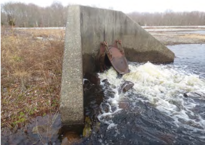
Figure 6.1.1c Segreganset River Pipeline Discharging into the Somerset Reservoir
