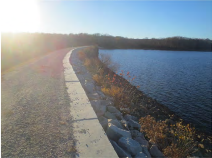
Figure 6.1.1a Somerset Reservoir Dam with New Crest
